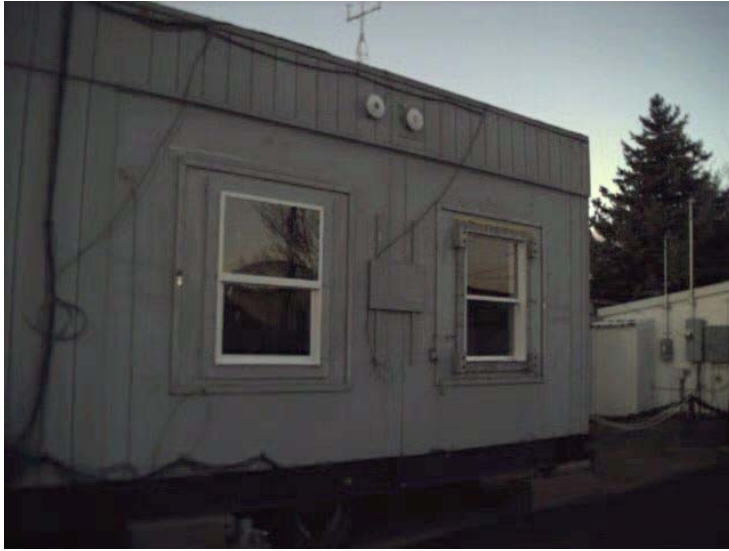
Figure 1. A View of the Test Facility. The faces of the two calorimeter chambers holding the test samples is shown. Left: Chamber B, holding the replacement window; Right: Chamber A with the prime/exterior storm combination. Also visible are the pyranometer and pyrgeometer (circular objects at top of wall, center) that measure the incident solar flux and sky temperature, and a portion of the weather tower (top, center) holding the wind speed and direction sensors.
